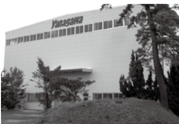
亀山工場の鋳造新工場 Newly built additional building for die cast production at Kameyama Factory
