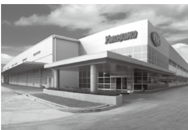
プラチンプリファクトリー新設 Newly built additional building at Thai Yanagawa Co., Ltd.
