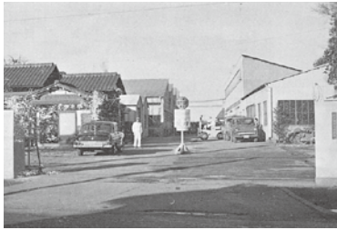
設立当初の府中工場 Fuchu Factory at its foundation
